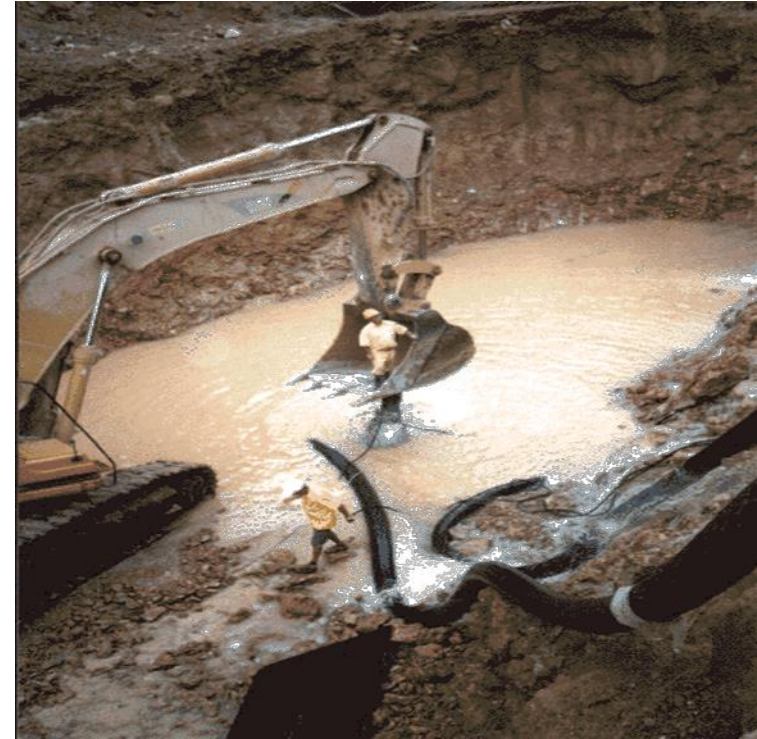
Straight Ground Water in During Excavation
